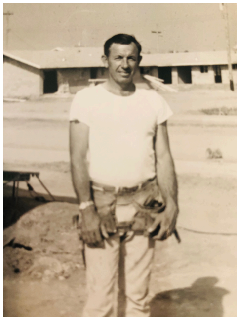
Housing construction in North Hanford
